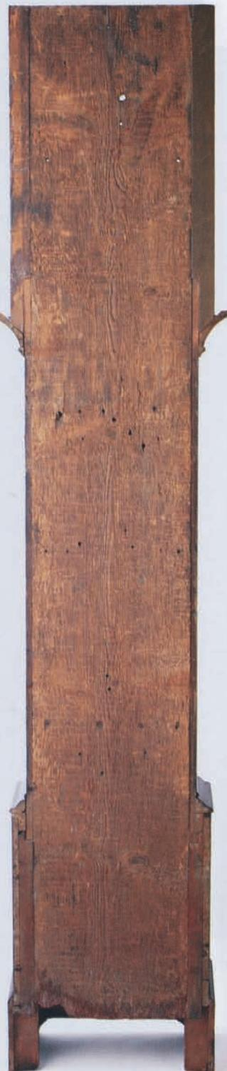
Pit-saw marks can be seen on the backboard of the case.
